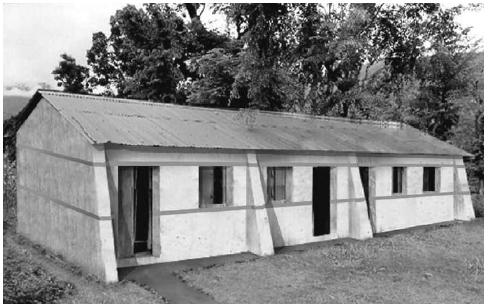
Figure 6-2 Buttress provide to exterior building
