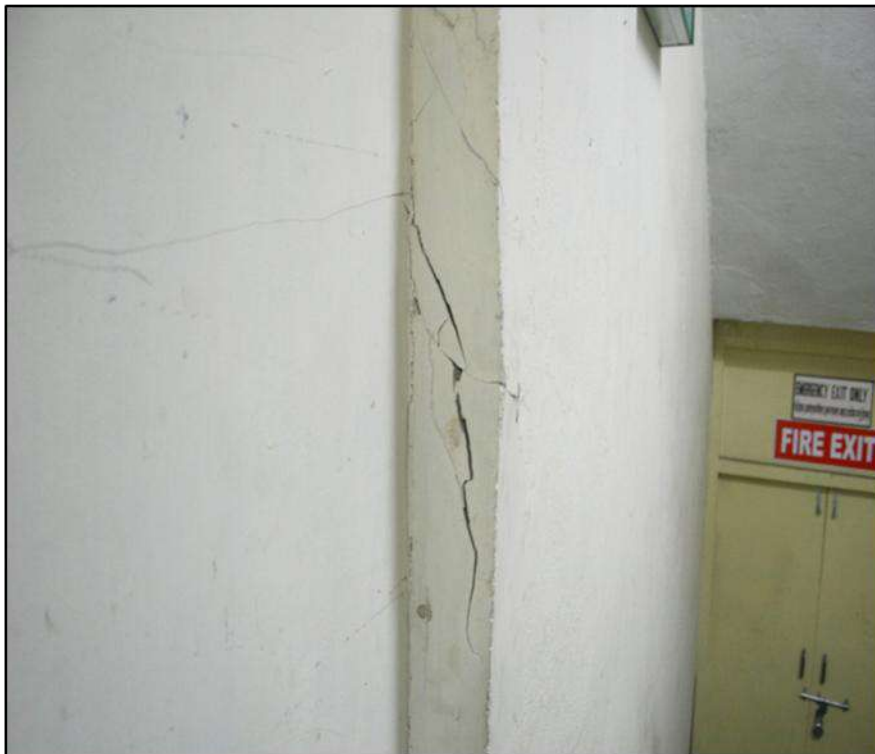
Figure 5-0-2 Damage grade 2 (source: MRB & Associates)
