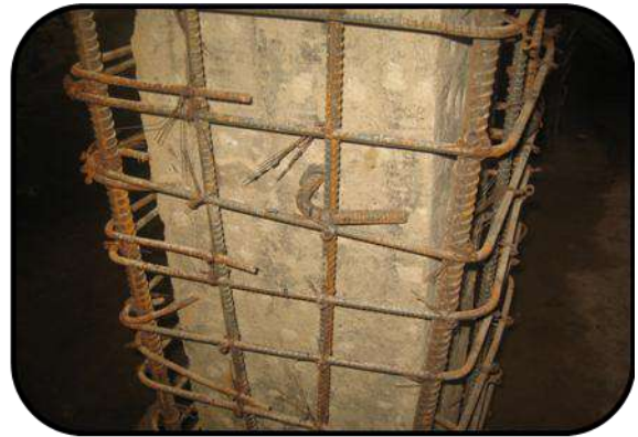
Anchorage of new reinforcement with the existing structure
