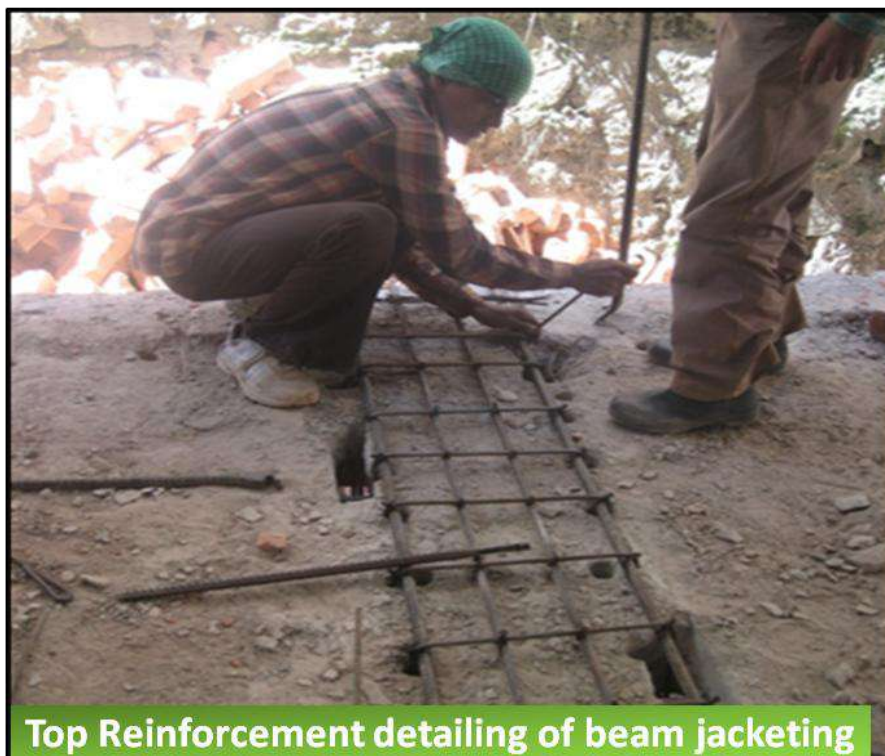
Figure 6-15 Top reinforcement detailing of beam jacketing
