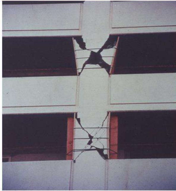
Short Column due to parapet wall
