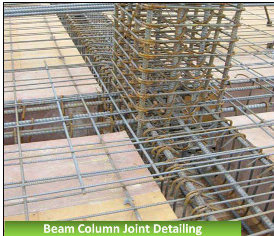
Figure 6-32 Beam column joint detailing (source: MRB & Associates)
