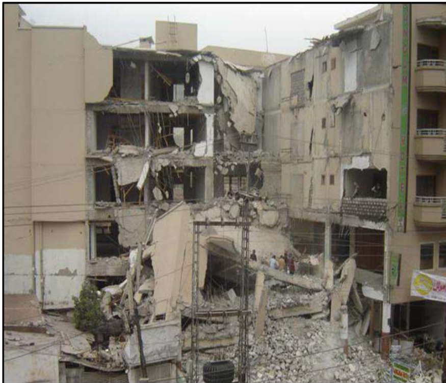
Figure 5-0-6 Damage grade 5 (source: MRB & Associates)
