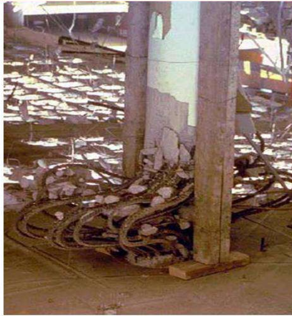
Column Tie spacing and hook
