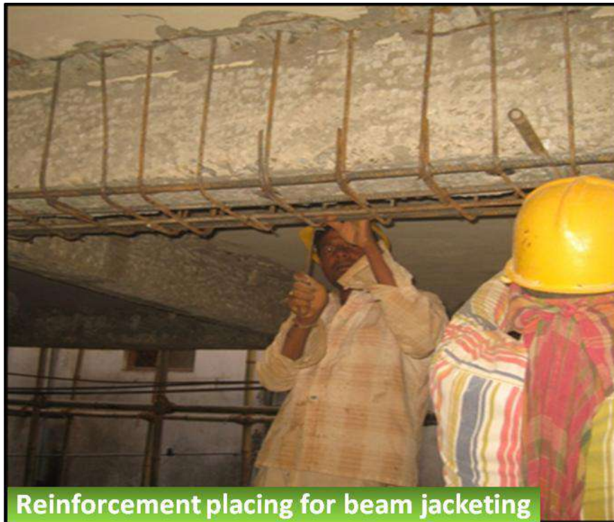
Figure 6-14 Reinforcement placing for beam jacketing
