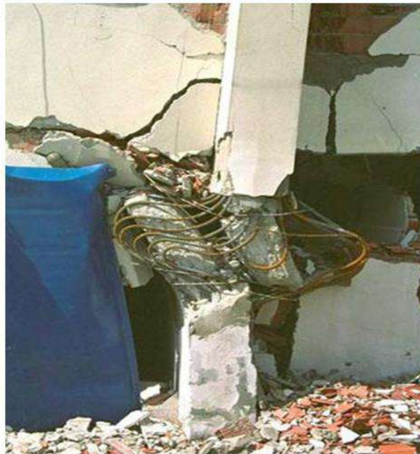
Column Tie spacing and hook
