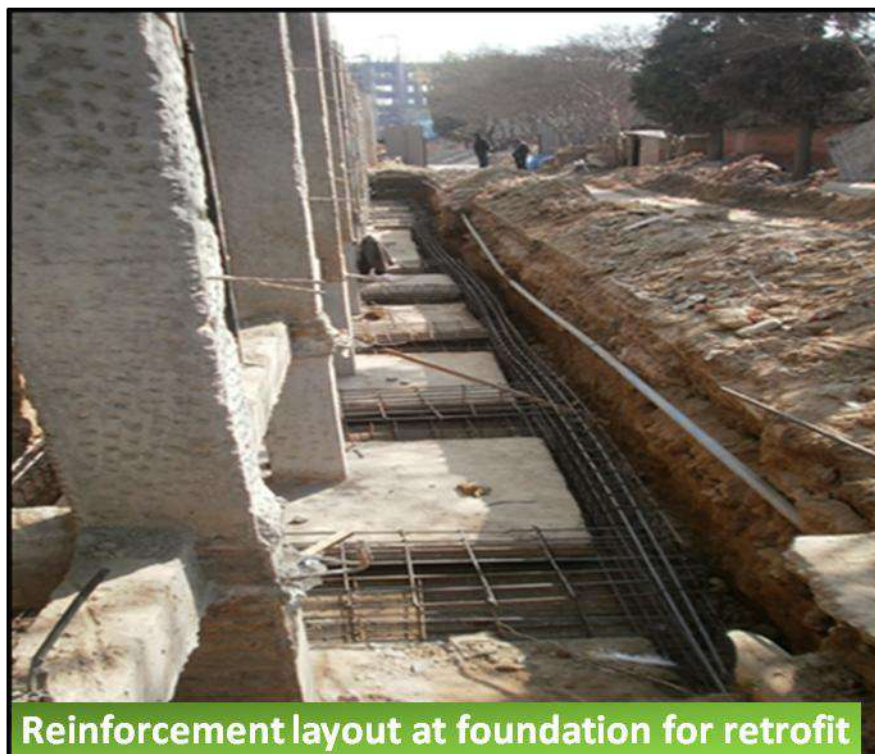
Figure 6-23 Reinforcement layout at foundation for retrofit (source: MRB & Associates)
