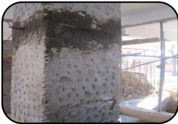
Roughening of old surface by chipping of existing concrete surface
