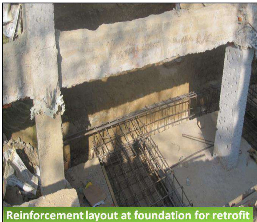
Figure 6-22 Reinforcement layout at foundation for retrofit (source: MRB & Associates)
