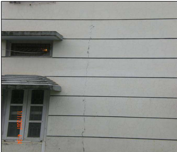
Figure 5-0-1 Damage grade 1 (source: MRB & Associates)
