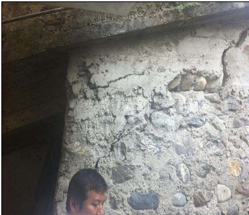
Figure 5-0-3Damage grade 3 (source: MRB & Associates)
