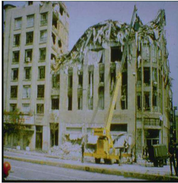
Damage due to torsion
