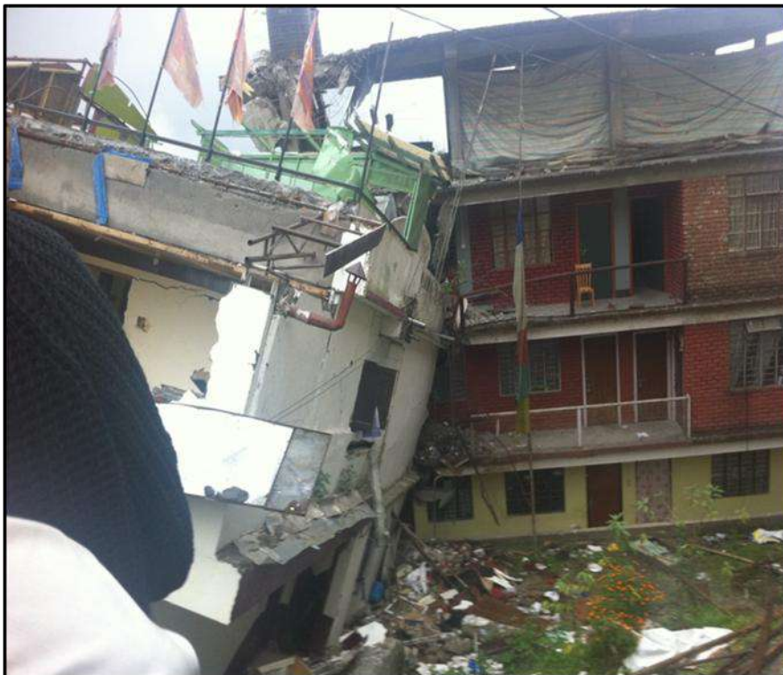
Figure 5-0-5 Damage grade 5 (source: MRB & Associates)
