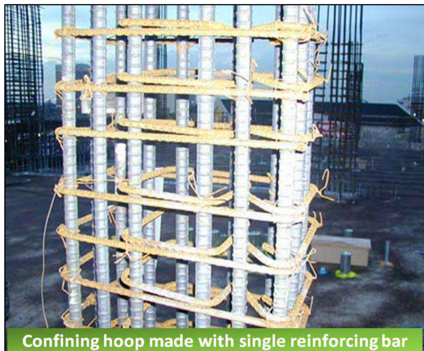
Figure 6-33 Confining hoop made with single reinforcing bar (source: MRB & Associates)
