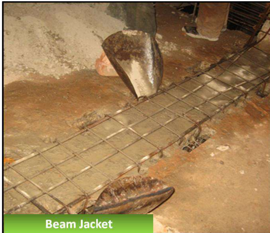
Figure 6-16 Beam Jacket (source: MRB & Associates)
