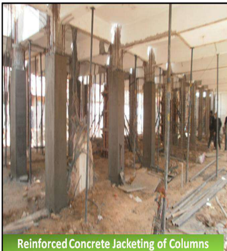
Figure 6-9 RC jackeing of columns
