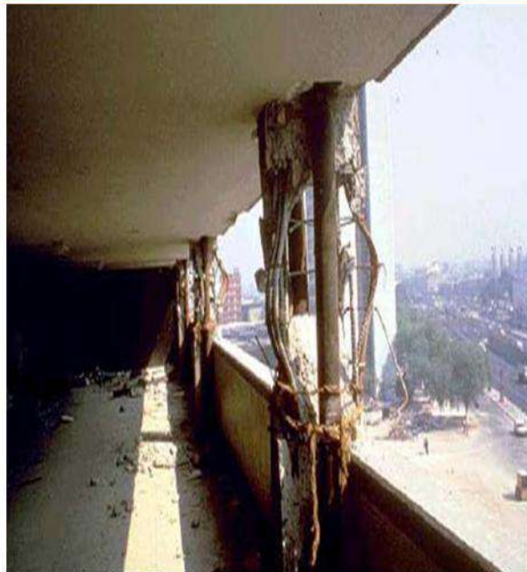
Short Column due to partial masonry wall
