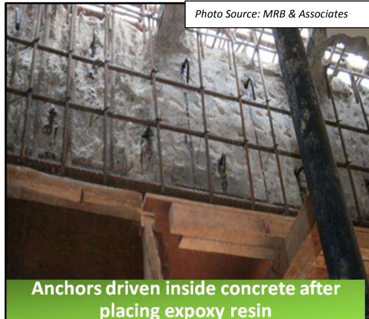
Figure 2-1 Anchors driven inside concrete after placing epoxy resin
