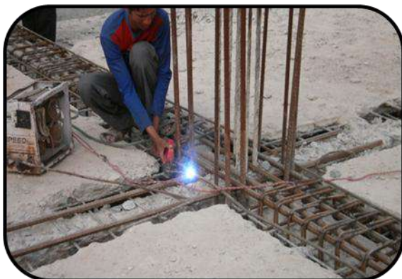
Welding of new reinforcement with existing one
