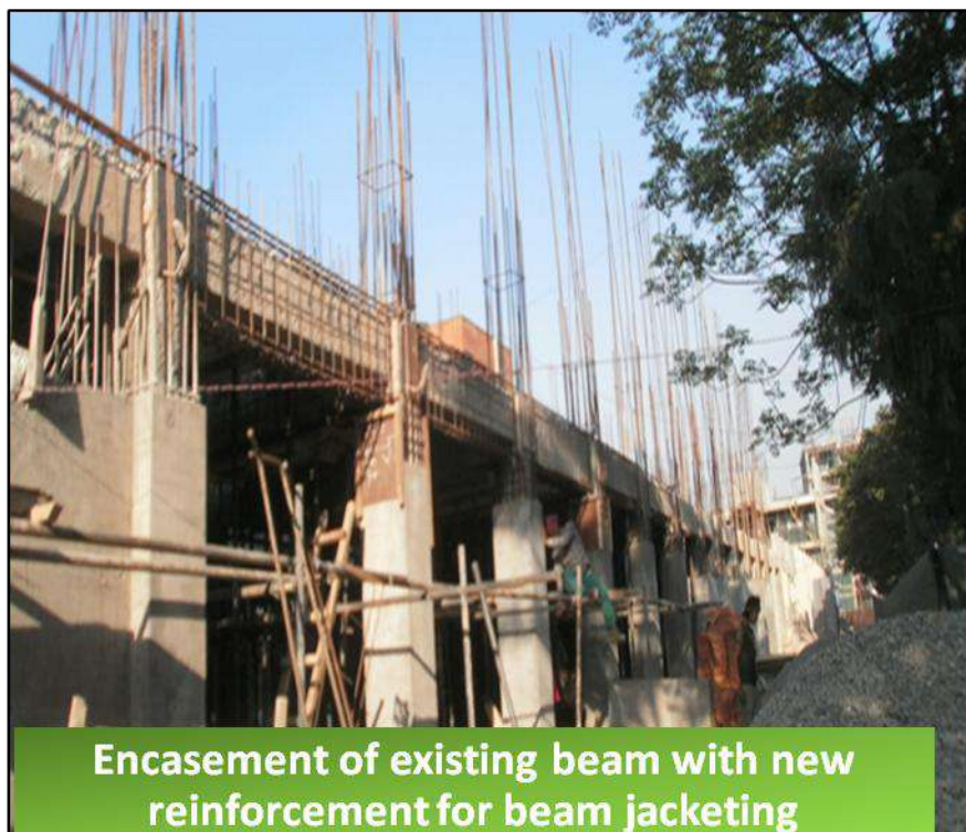
Figure 6-17 Encasement fo existing beam (source: MRB & Associates)
