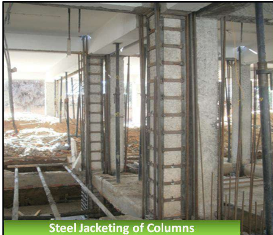
Figure 6-11 Steel jacking of columns (source: MRB & Associates)
